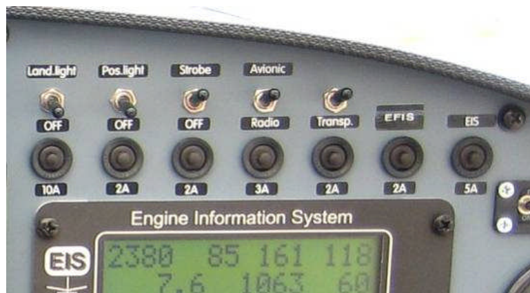
Figure 7 – Switches and fuses panel (older panel shown...)
